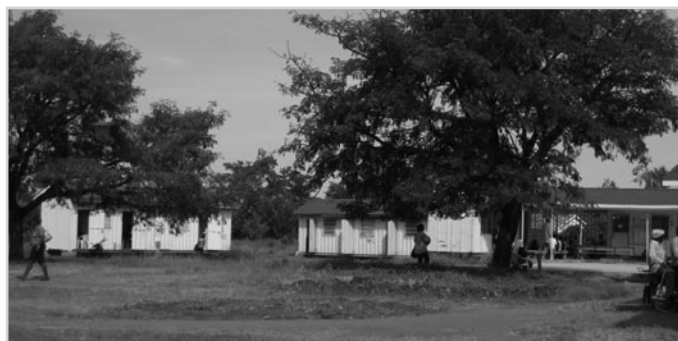
Picture 2: An HIV clinic in a rural area of Kenya, built using old shipping container boxes, part of the community health centre.
